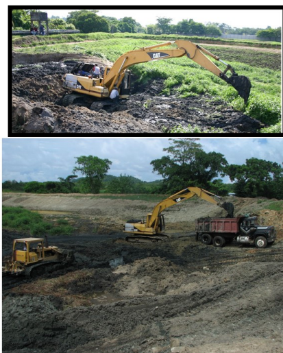
Figure 6. Waste stabilization pond sludge removal from waste stabilization pond in Tela, Honduras. In the upper photo an excavator removes surface and deep sludge (up to 1 m) from pond planted with deep root wetland plants. In total, 3,000 m 3 of dried sludge was removed in 5 days with the excavator (after pond was dried by draining and planting of deep rooted wetland plants) (photos provided by Stewart Oakley with permission).
