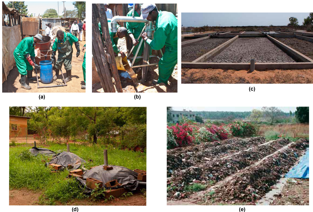
Figure 9. a) Transport of fecal sludge from an informal settlement in Nairobi. b) Addition of water to pit latrine to aid removal of pit contents in Nairobi, c) drying bed for treatment of fecal sludge in Dakar, d) biogas reactors used to stabilize fecal sludge in Ouagadougou, (photos (a-d) provided by Linda Strande with permission) pilot composting facility that combines fecal sludge and municipal solid waste in Bangalore (photo (e) provided by Christian Zurbrugg with permission).
