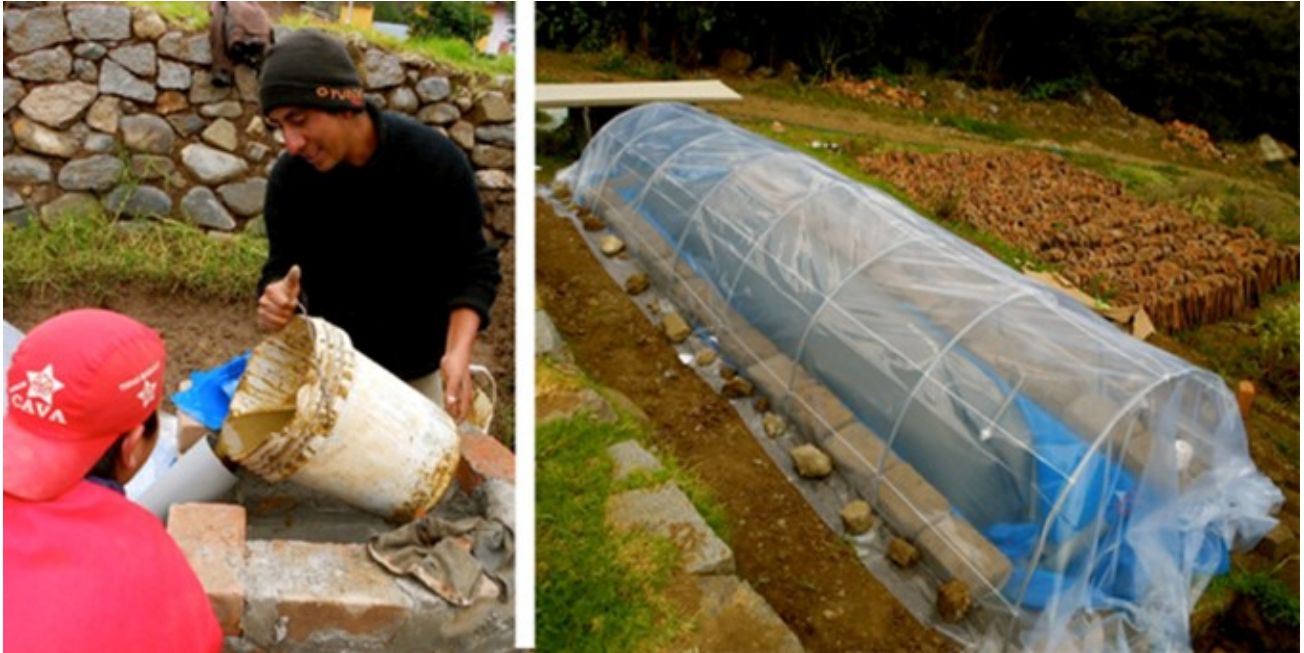
Figure 3. Left) Filling a tubular anaerobic digester with sludge. Right) Tubular digester (dark cylindrical tube) located inside a clear plastic covering to promote higher temperature (photos provided by Danielle DeVuyst with permission)
