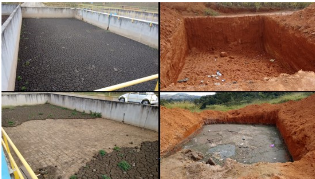
Figure 10. Example of safe management of sludge in a small town in southern Brazil with sludge drying beds (upper left), emptied manually by personnel using protective equipment (lower left); dried sludge is then buried onsite in pits (upper and lower right) (photos provided by Matthew E. Verbyla with permission)
